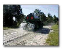
Figure 11. Water truck applying dissolved polymer flocculant
