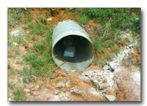
Figure 39. Polymer block in a construction site culvert
