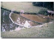
Figure 30. Particle curtains clarifying the input to a pond
