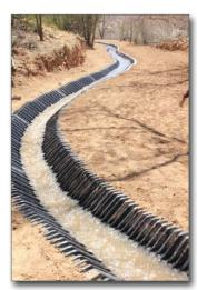
Figure 18. In-ground treatment ditch
