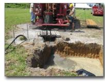
Figure 7. Drilling rig and settling pit
