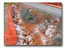
Figure 38. Eroding gully on a construction site
