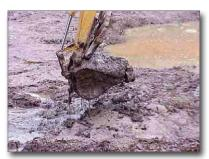
**Figure 36.** Removing stiffened sediment from a sediment basin
