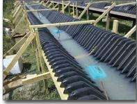
Figure 17. HDPE treatment ditch liner
