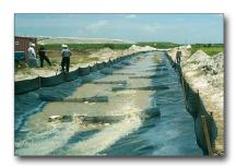
Figure 16. Flocculation ditch with checks to increase the polymer mixing
