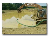
**Figure 14.** Sediment basin to be dewatered
