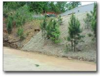
Figure 4. Slope covered with floc collection matting
