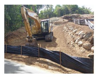
said, the silt fence incorrectly installed in the photo to the right is an indication that this permittee doesn't understand and/or appreciate the vital importance of NPDES Permit compliance for protecting America's future; and more specifically, the potential road hazard and water quality problems in the creek adjacent to this project. Site inspections are only part of BMP compliance, documented maintenance must follow!
