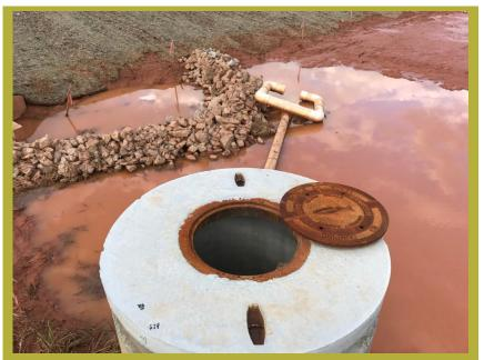
As in the photo above, the filter ring may also be placed below storm drains that discharge into detention ponds, creating a centralized area, or "forebay", for sediment ac cumulation. This provides for easier, more localized clean-out of the pond.
