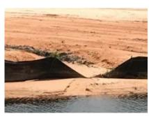
Recent rains have produced high volumes of sediment which is overwhelming poorly installed silt fences, causing wood posts to come out of the ground and the fabric to detach from the posts. In areas where the slope is
